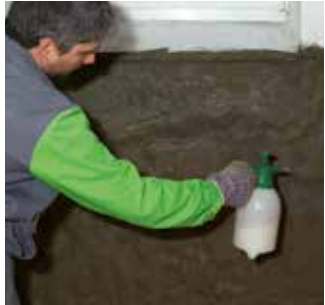
Priming with KÖSTER Polysil TG 500
