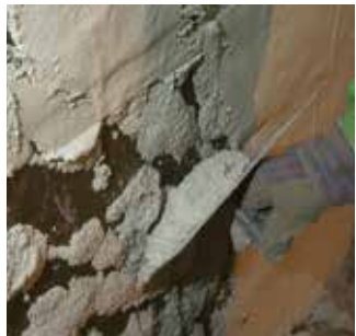
Application of KÖSTER Restoration Plaster
