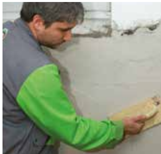
Floating the surface
