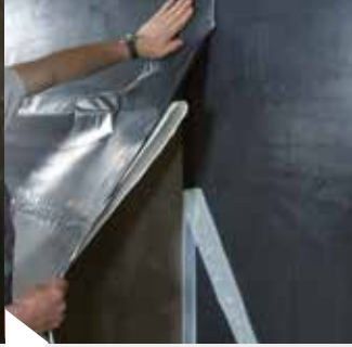
Applying the membrane
