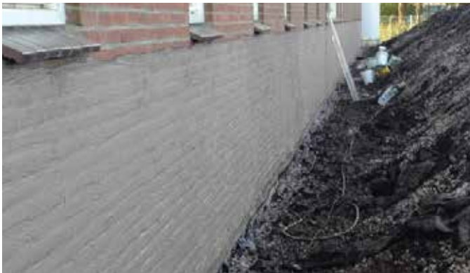
External basement waterproofing
