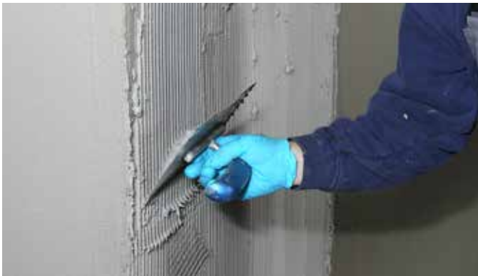
Internal basement waterproofing
